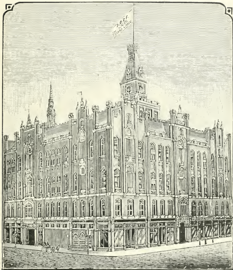
I. O. O. F. BUILDING, SEVENTH AND MARKET STS. San Francisco, Cal.
